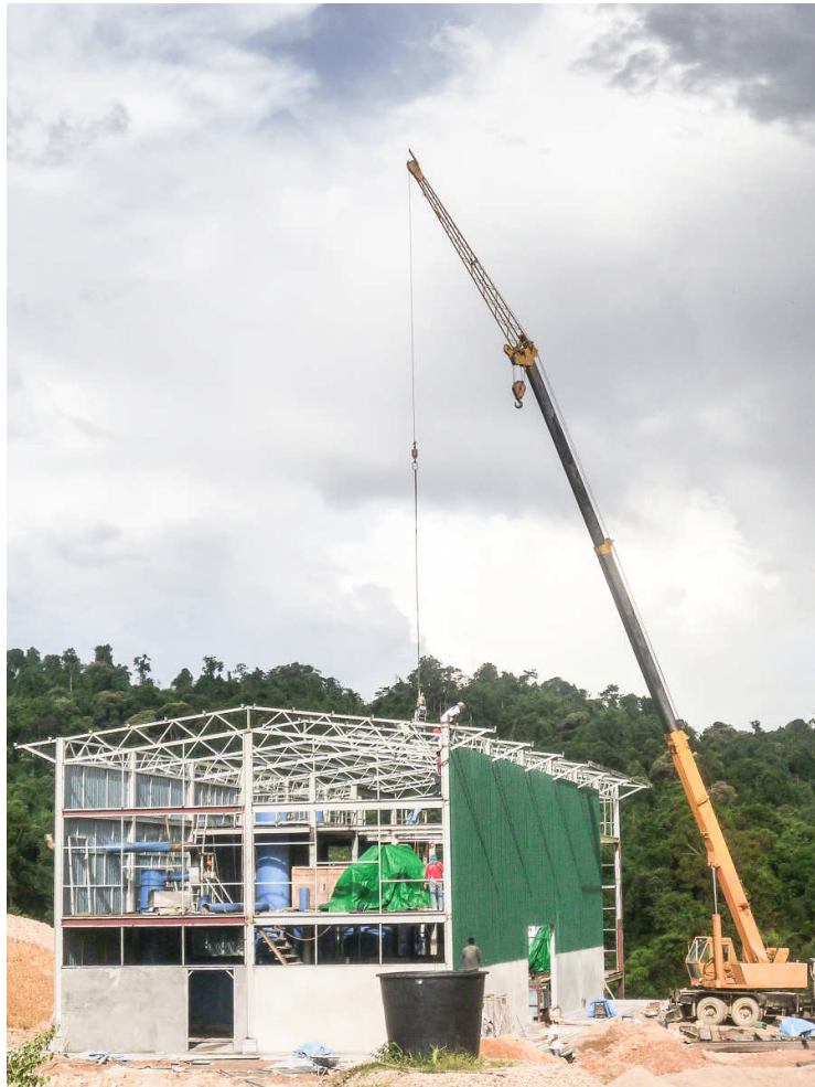
CNMC Photo: Construction of the second gold de-absorption processing plant.
