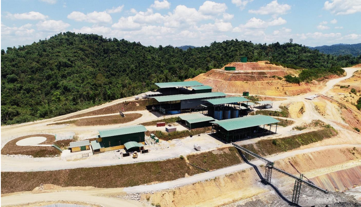
Figure 3.2 Sokor CIL plant and tailings facility – March 2019
