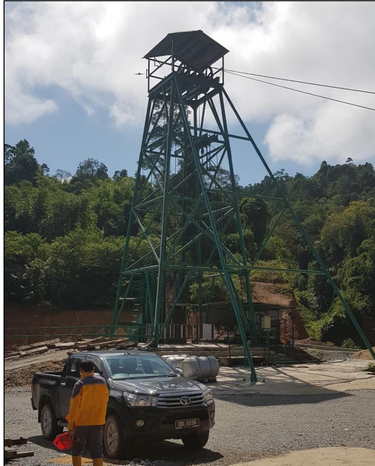
Figure 3.4 Ketubong shaft headframe – October 2019
