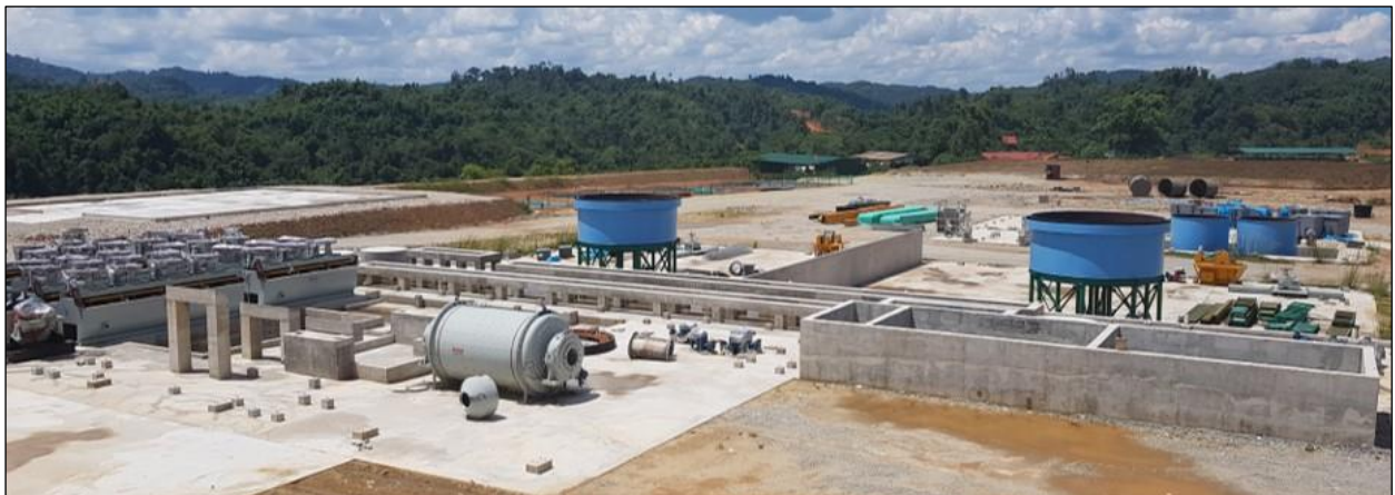
Figure 3.3 Construction of Sokor flotation plant – October 2019
